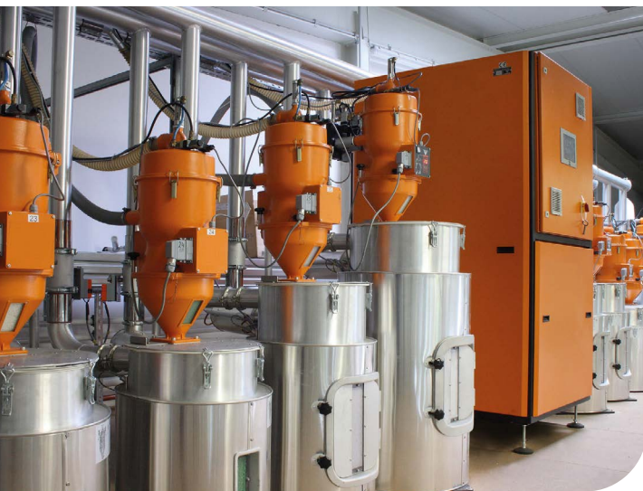
Suction & transport hoses used for filling granule dryers along with temperature-proof hoses for transporting the air for the dryer itself
